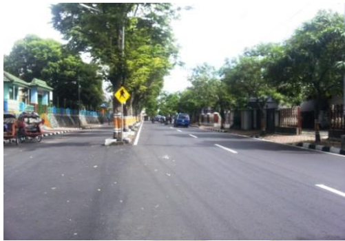
Figure 2. Existing Condition on Jalan Pahlawan
