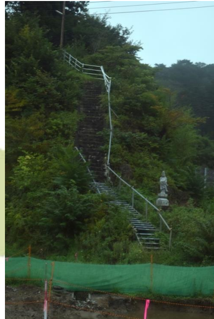
Figure 23 Escape stairs toward the top of the hill
