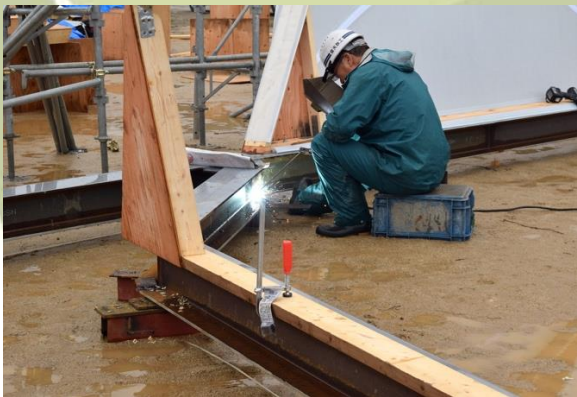
Figure 12 Welding the foundation components
