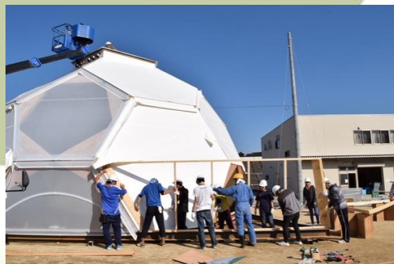
Figure 19 Construction of extended room
