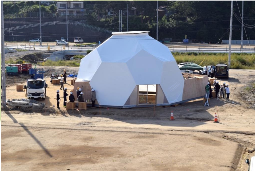
Figure 1 The final stage of Odense 3 dome construction
