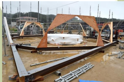
Figure 17 Assembly of wall components on the steel foundation
