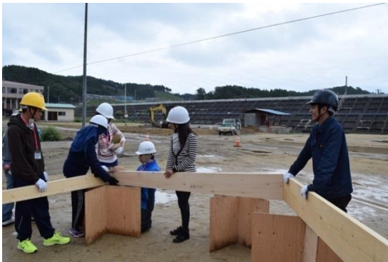
Figure 14 Construction of pentagonal and hexagonal wall frames
