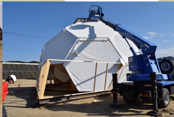
Figure 13 Operating the mobile crane
