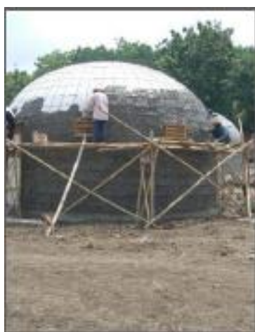
Figure 20. Casting concrete monolith. (Source: DFTW, 2008)
