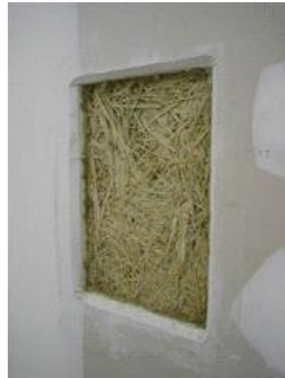
Figure 3b. Two layers of paddy-straws panels was put side by side, the tiny cavity gap between panels and wall were filled with rock wool floss to sealed it
