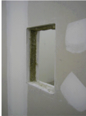
Figure 3a. Hole of dimension of 400 mm x 300mm was made on the existing filler wall (i.e. gypsum walls)
