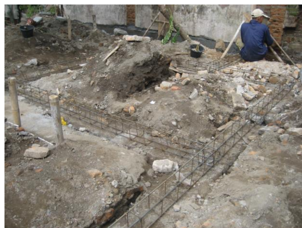
Figure 2. Building reinforcing steel bars
