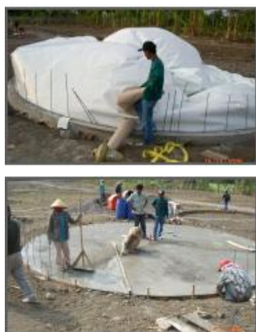
Figure 19. Casting molds and preparation of concrete floors balloon (Source: DFTW, 2008)
