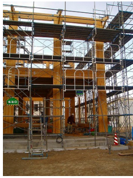
a) Glulam school class room under construction
