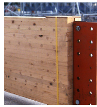
a) Prefabricated beam with concealed steel gusset plate and drift pins.
