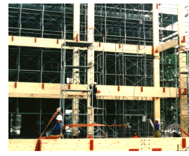
b) On-site assembly of glulam three story portal frame.
