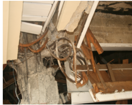
b. Damaged beam-column joint
