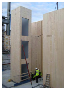
a) On site assembly of wall element made of CLT panels having openings already processed in the factory.(Courtesy of Mr. Matti Linegar)
