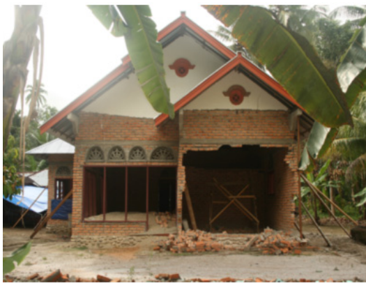
a. Improper built house in Padang Pariaman
