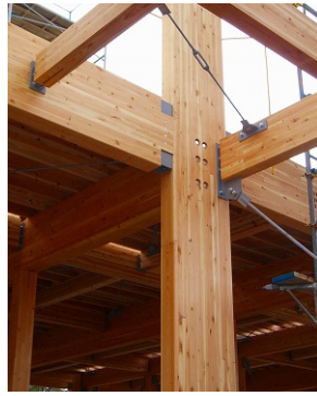
b) Details of beam-column joint
