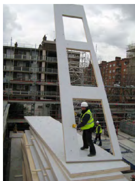
a) On site assembly of wall element made of CLT panels having openings already processed in the factory.(Courtesy of Mr. Matti Linegar)
