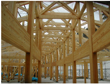
a) Glulam frame structure under construction
