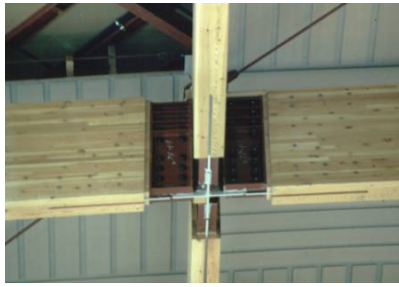
a) Two ways joint before completion
