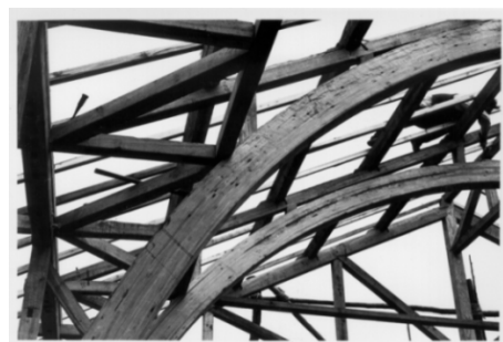
b) Details of glulam arch structures.
