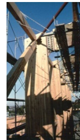
c) Assembled beam-column joint
