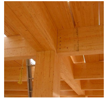
c) details of beam-column joint
