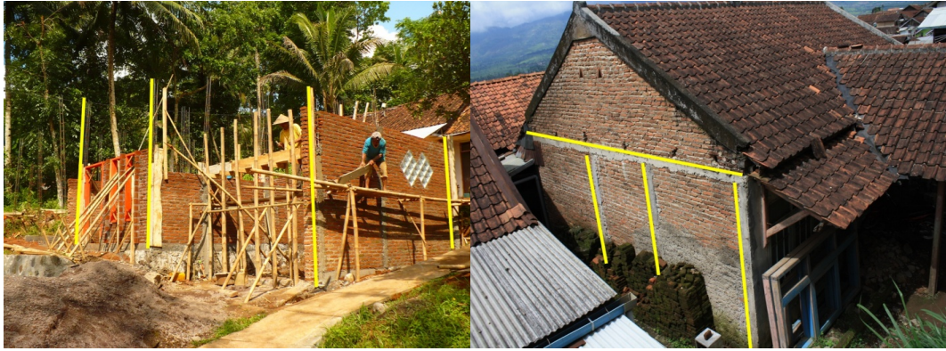
Figure 2 Reconstruction Process of Earthquake-Resistant Housing. Picture Information (left to right): One of the housing reconstruction process in Panjalu District which has implemented the using of column (Source: Observations, 2010); House in the Pangalengan District which have applied one part of technical guides of earthquake resistant construction (Source: Observations, 2012).
