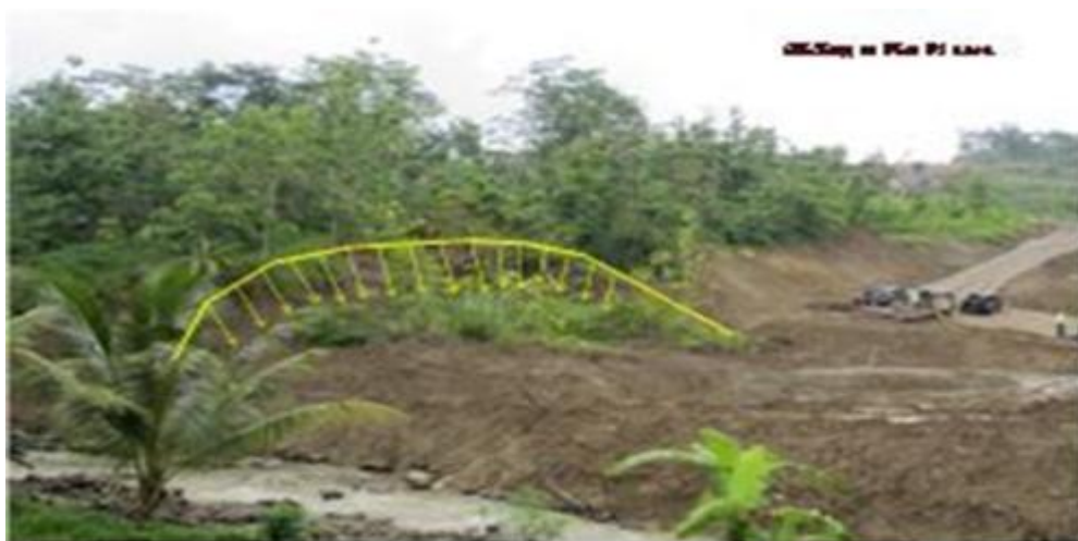
Figure 3. Slip Failure at Slope beside the Pier P1 structure (1)
