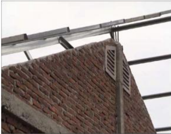
(a) No reinforced concrete roof band
