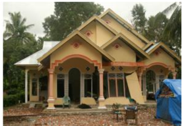
(b) Un-reinforced masonry brick wall
