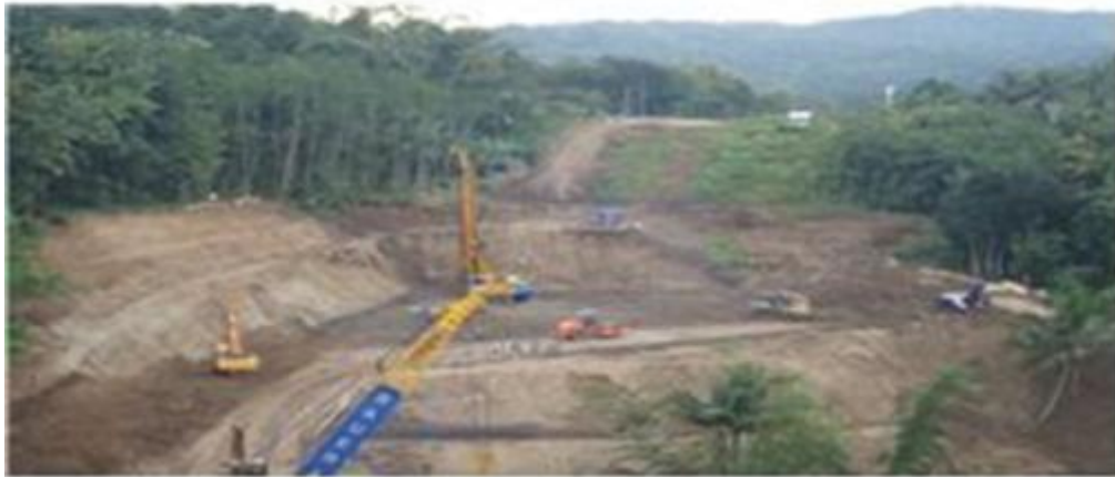
Figure 3. Slip Failure at Slope beside the Pier P1 structure
