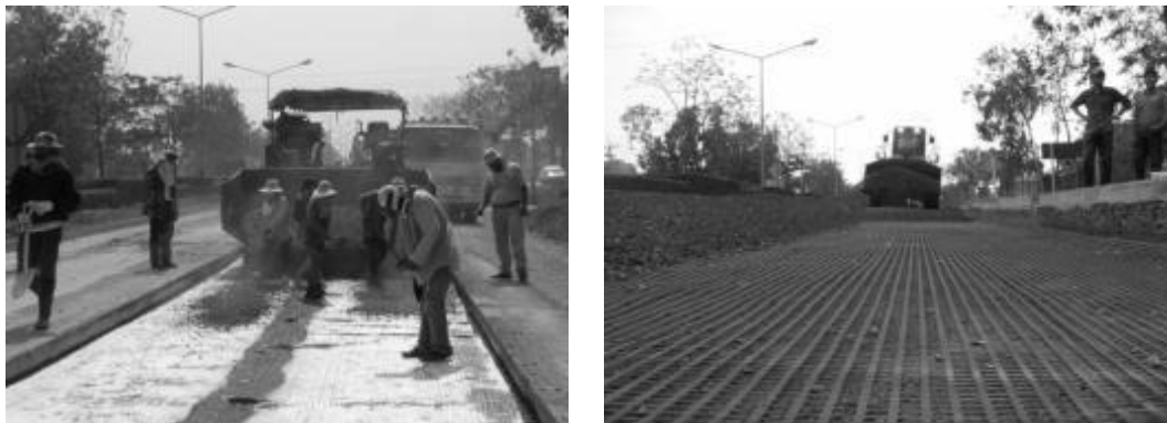
b) Geogrid reinforced pavement
