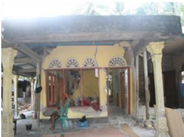
(a) Improper reinforced concrete canopy
