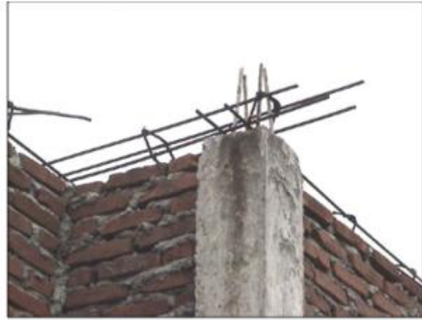
(b) Poor ties, rebar detailing and no hook at joint
