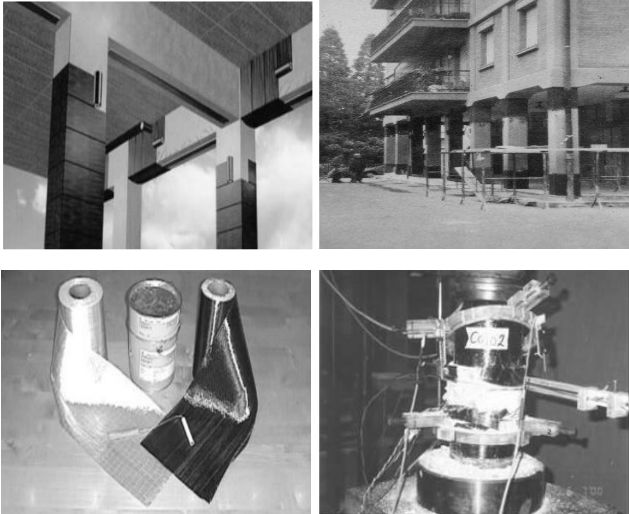
Figure 5. Use of FRPs as externally bonded reinforcement
