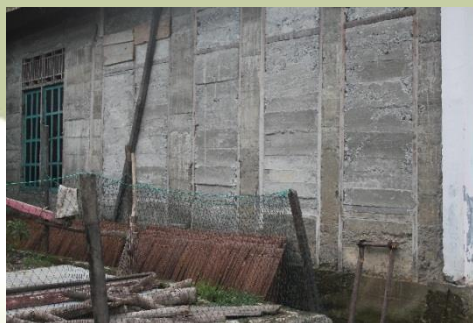
Figure 4 Walls Construction with Concrete Casting Technique
