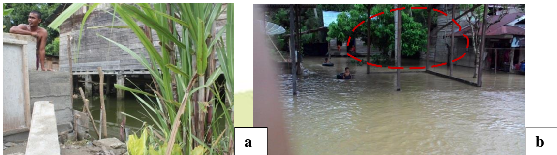
Figure 2 a. On the condition of flooded land, there are two different home constructions, the stilt construction and the construction on the ground; b. Research Area in flood conditions. The flood waters do not reach the floor of a stilt house
