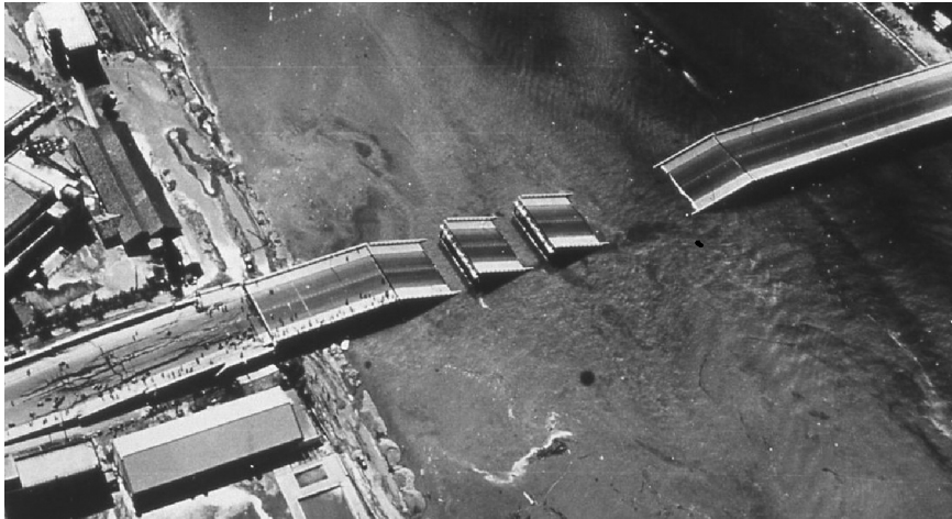
Figure 3. Showa Bridge failure due to 1964 Niigata earthquake and liquefaction phenomenon (Kerciku et al 2008) [13].
