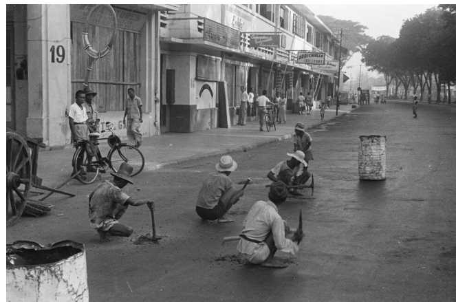
Figure 2. Jalan Veteran 1948, Perbaikan jalan pasca Kemerdekaan RI Source: https://www.lostjakarta.com/tag/citadelweg
